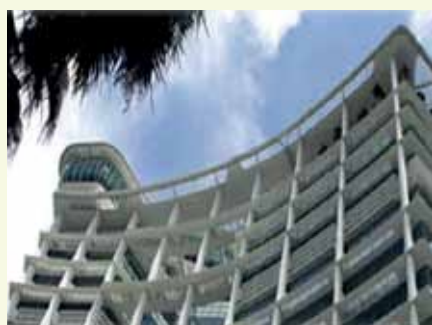
Light reflectors cut down on the need for indoor lighting.
